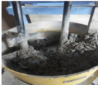
Fig 3.11: Mixing of Concrete
