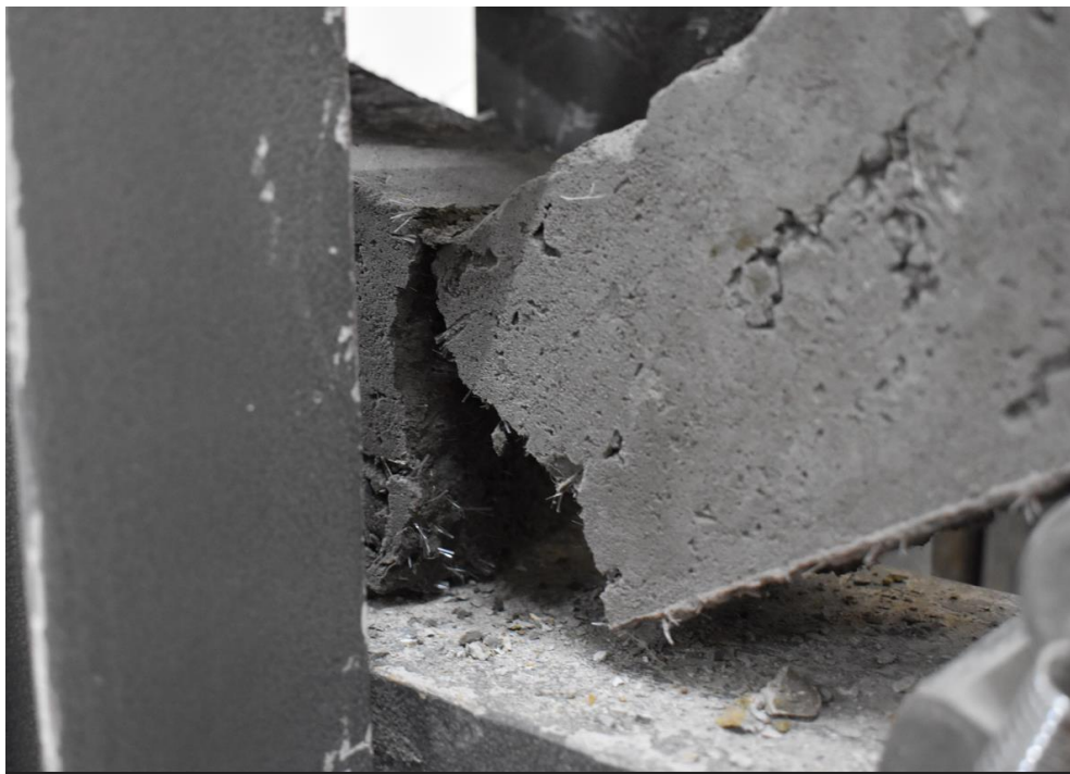
Fig 3.13 Testing of beam in flexure testing machine
