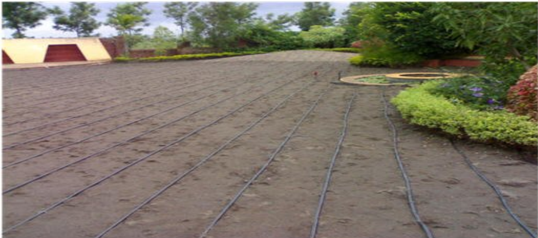
fig 7.2 : Installation of subsurface land irrigation system
