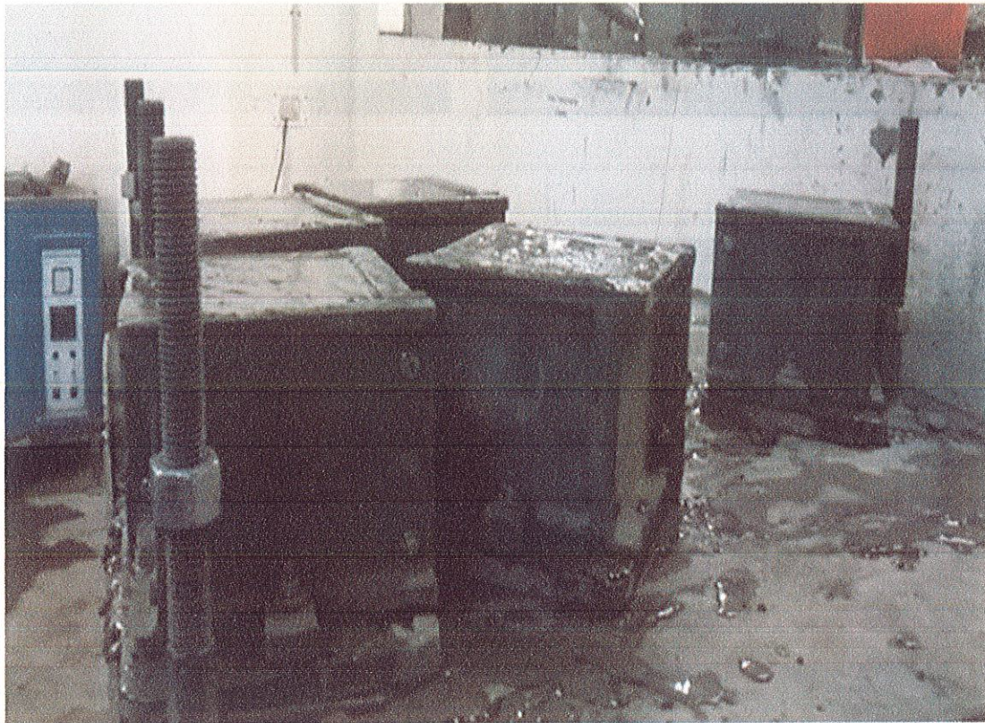
Picture 6.4 : Compaction using vibrators
