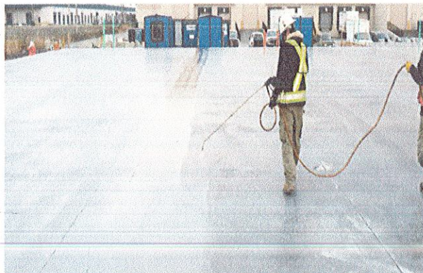
Picture 2.2 : Spraying of curing compounds
