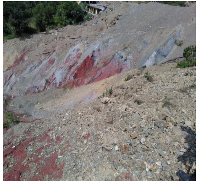
Fig. 1: Section of Kotropi (Mandi, Himachal Pradesh) landslide
