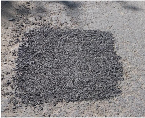
Fig. 4: Patching at RR-1
