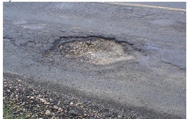
Fig. 3: Pothole Depression
