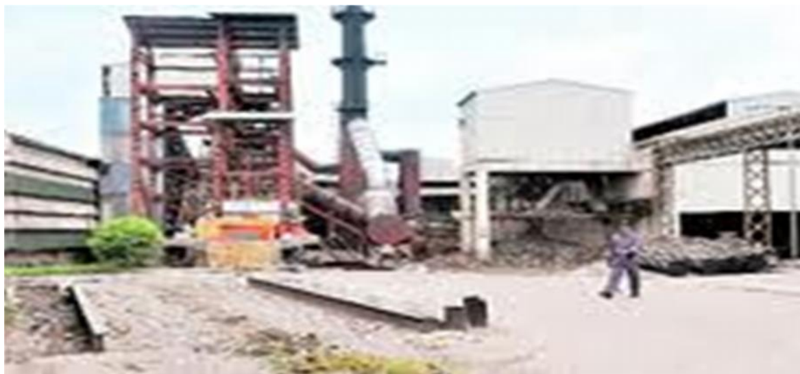
Figure 5: A view of plant
