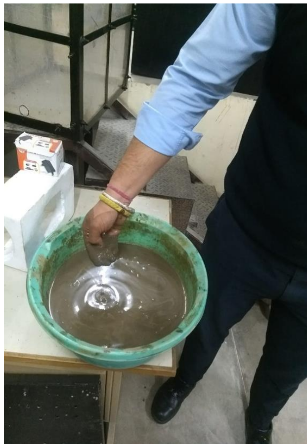
Fig. 3.19 Preparing BCS Grout
