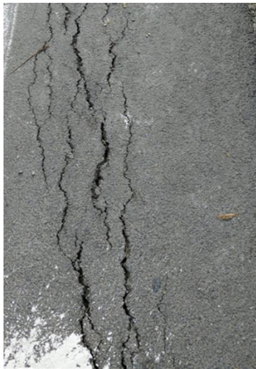
Fig.4.7: Longitudinal cracking at RR-1
