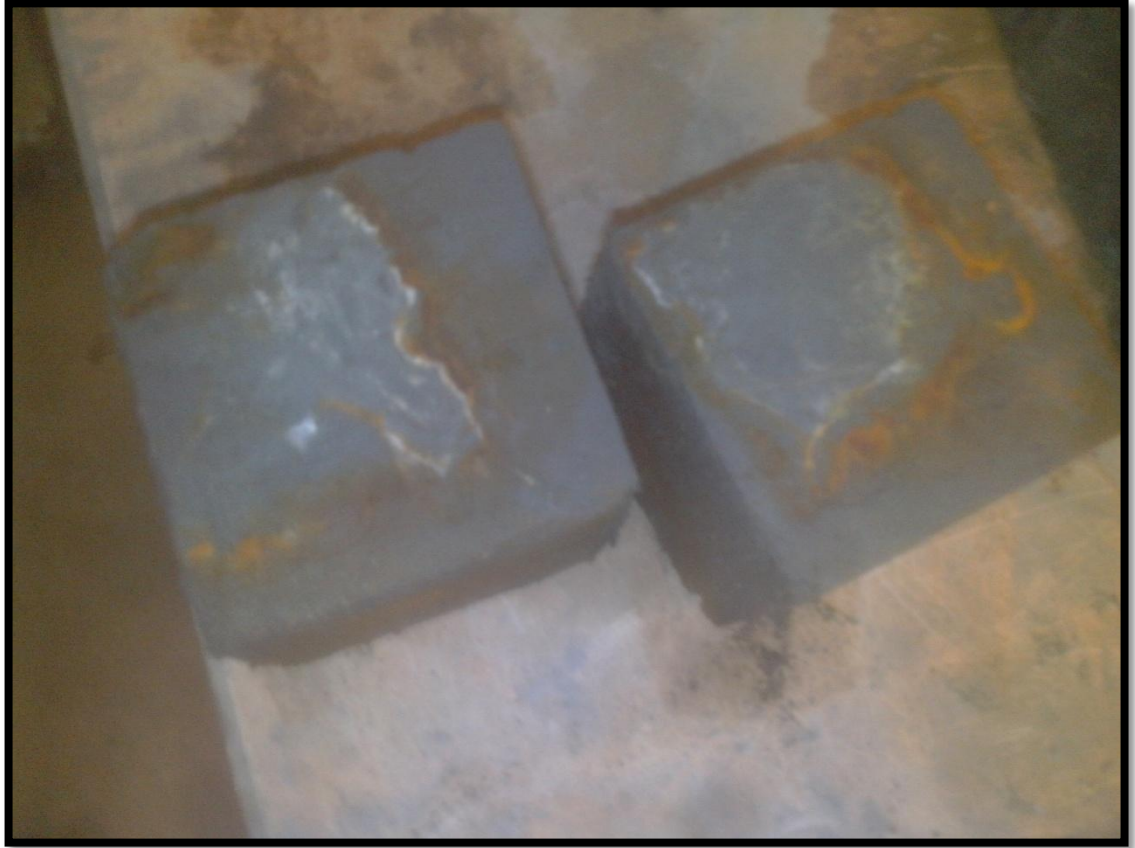
Figure 3.11 Condition of cubes after 21 days exposure to 5% HCl solution
