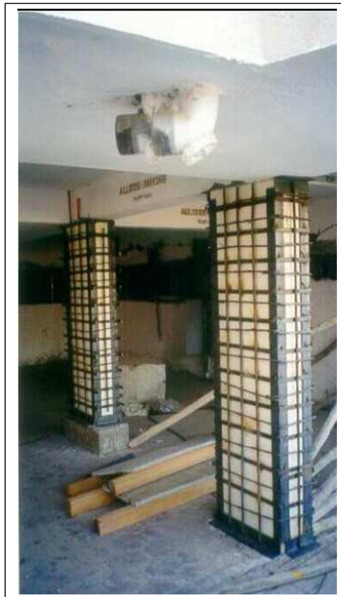
Fig 1.2: Steel Jacketing
