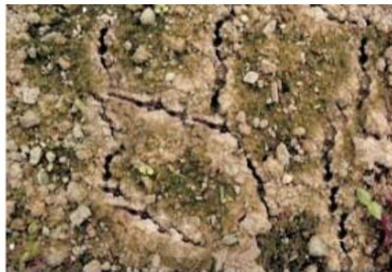
Fig.1. Typical Cracks in Black Cotton Soil in Dried State Picture Reference—( www.ijera.com )
