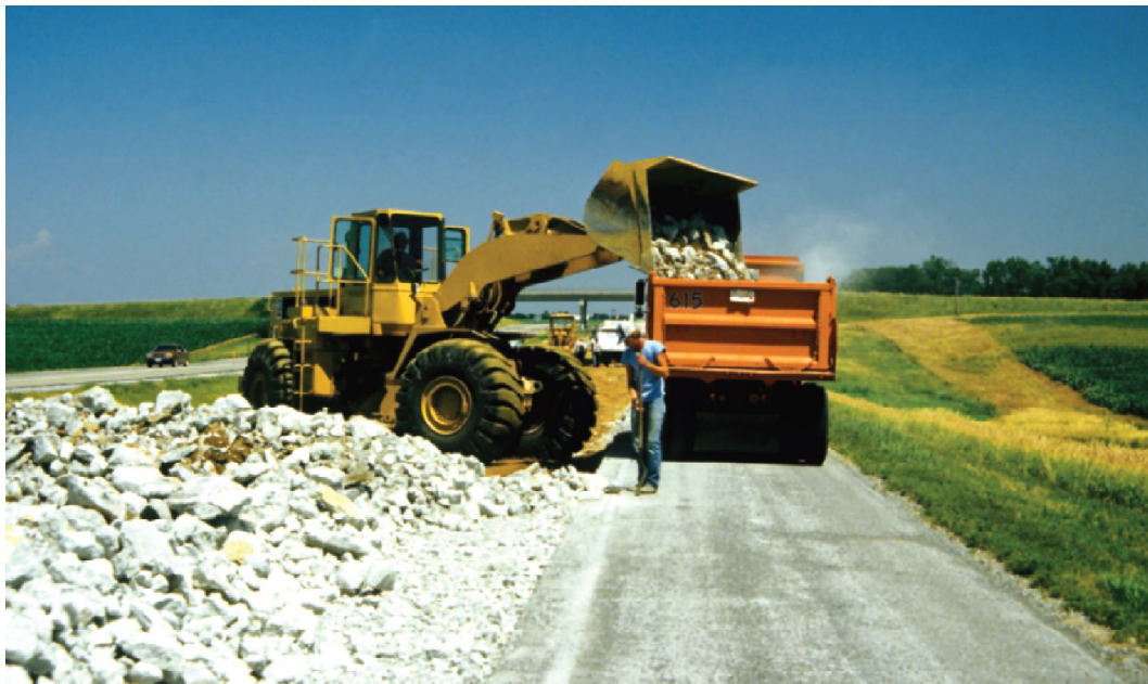
Figure 4.2 - Front End loader
