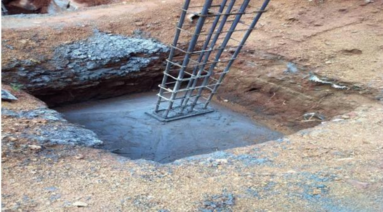
Fig 2 –footing of column
