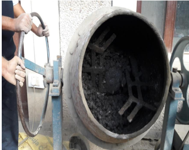
Fig 3.7. Concrete mixture in mixer
