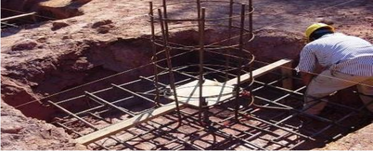
Fig.14: Isolated Footing Reinforcement
