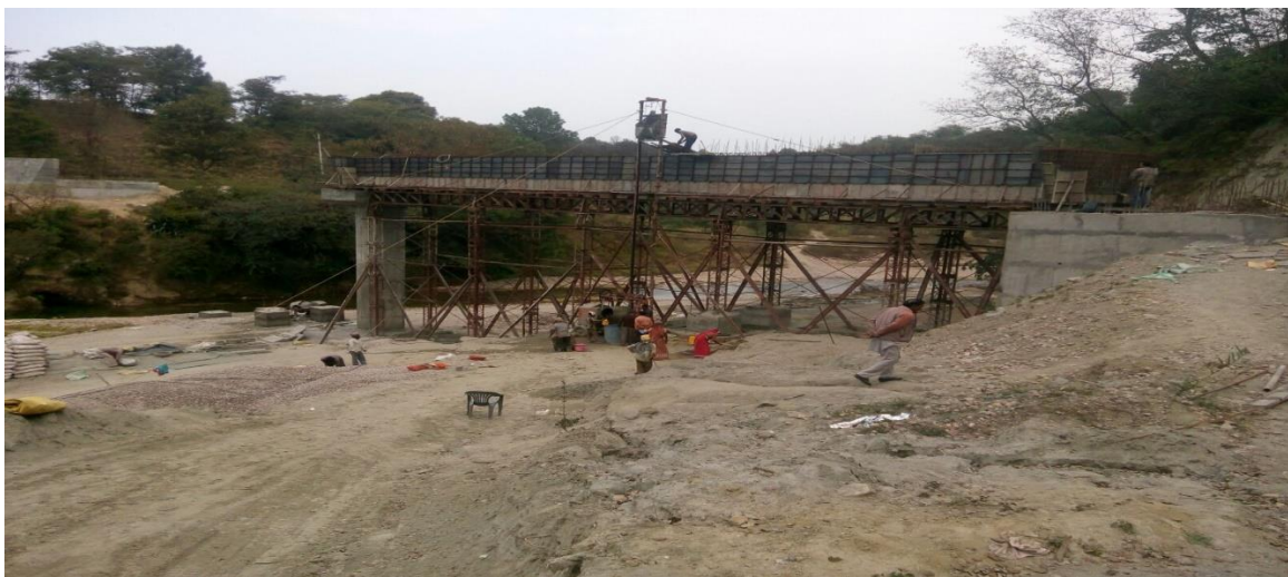
Fig. No 1.1 Saheli side span of bridge over Man Khad
