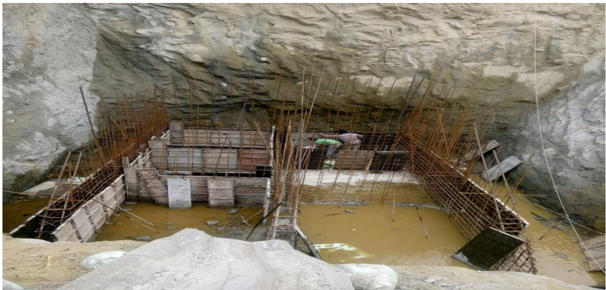
Fig No 1.4 Saheli Side Abutment
