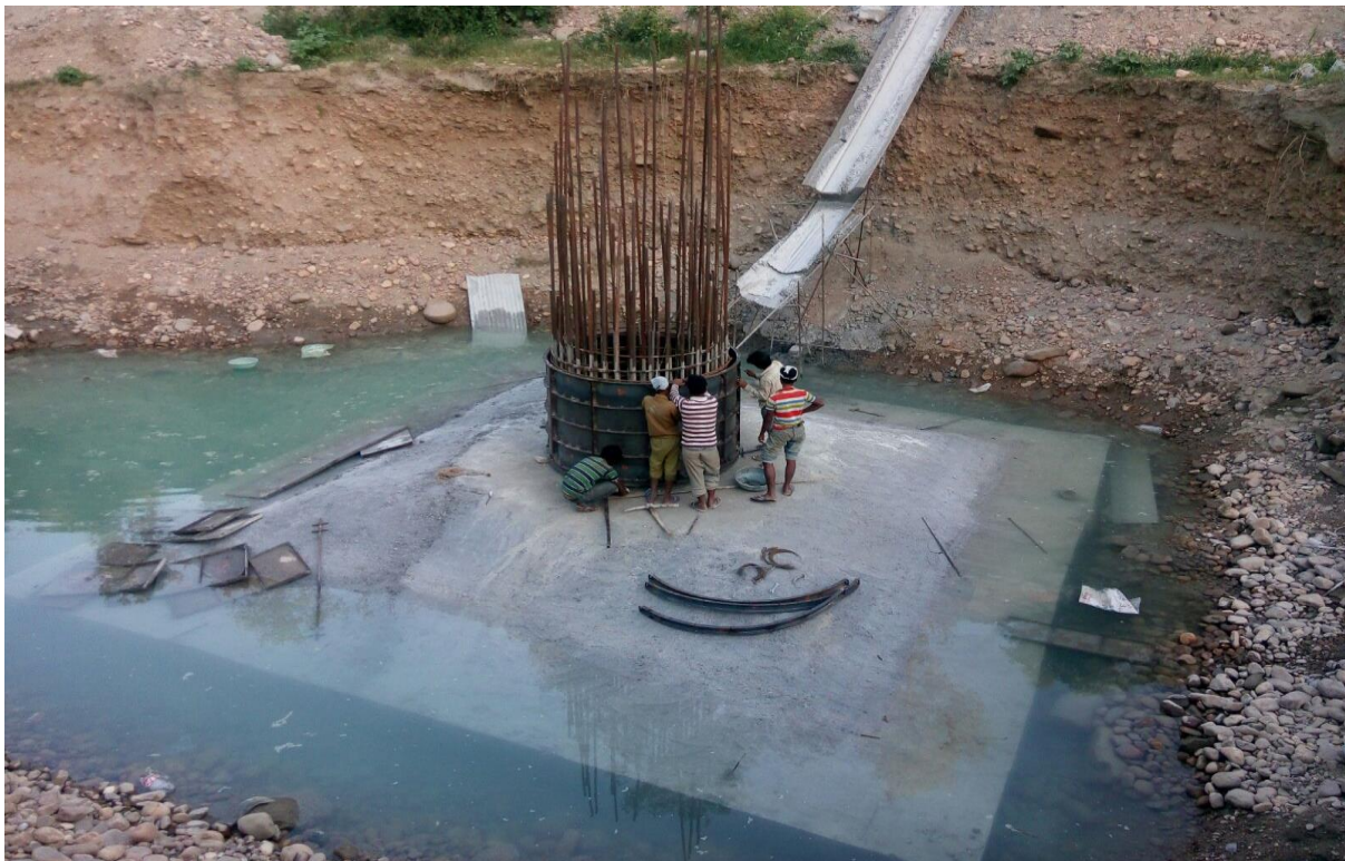
Fig.No 1.2 Raft foundation of Pier
