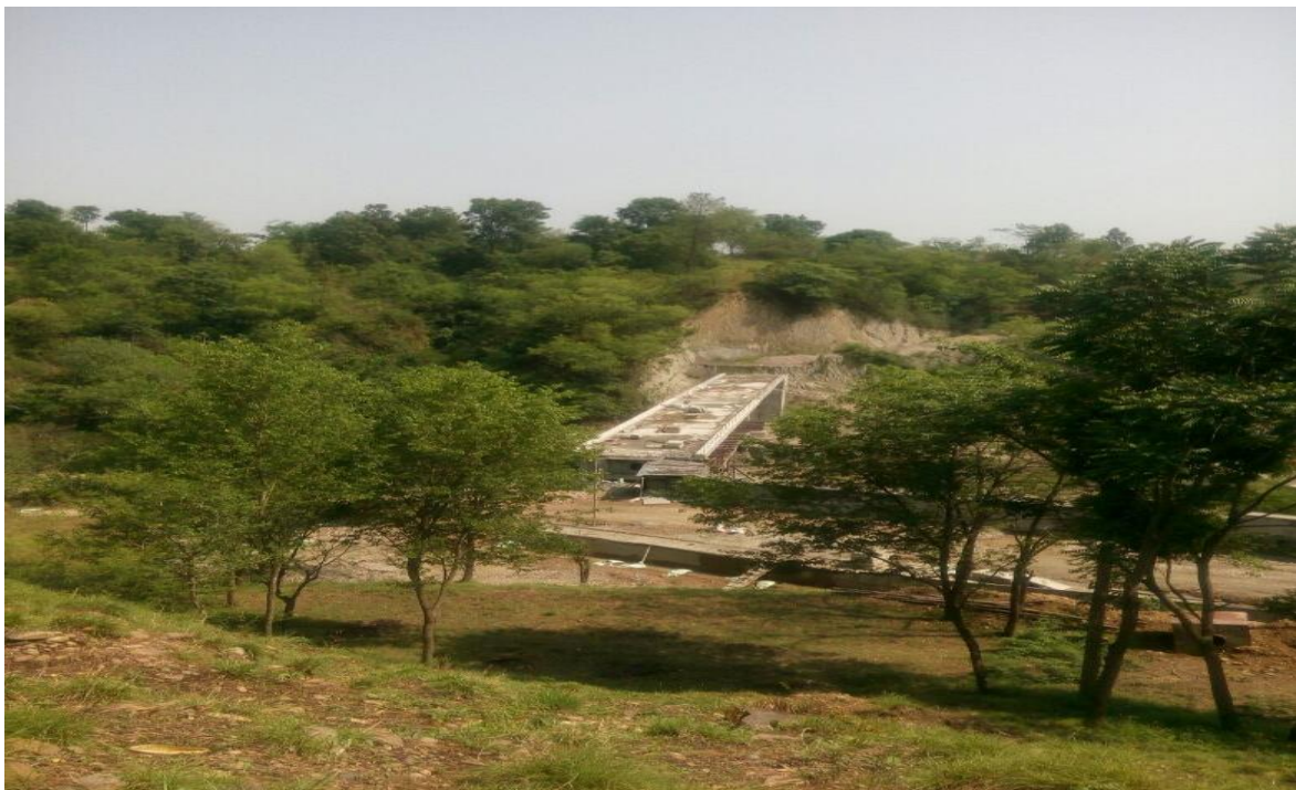
Fig. No 1.5 Slab of bridge
