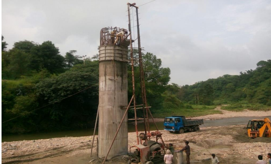
Fig No 1.3 Pier of the Bridge
