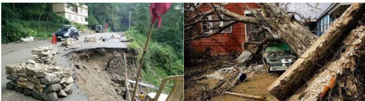
Figure 8.3: Damage caused by Landslide and Earthquake.
