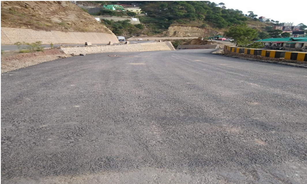
Fig 4.1 Laying of Flexible Pavement on Site
