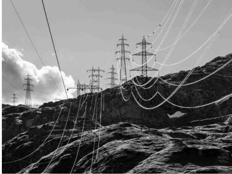
Fig 3.1: Sagging of Guy Wires
