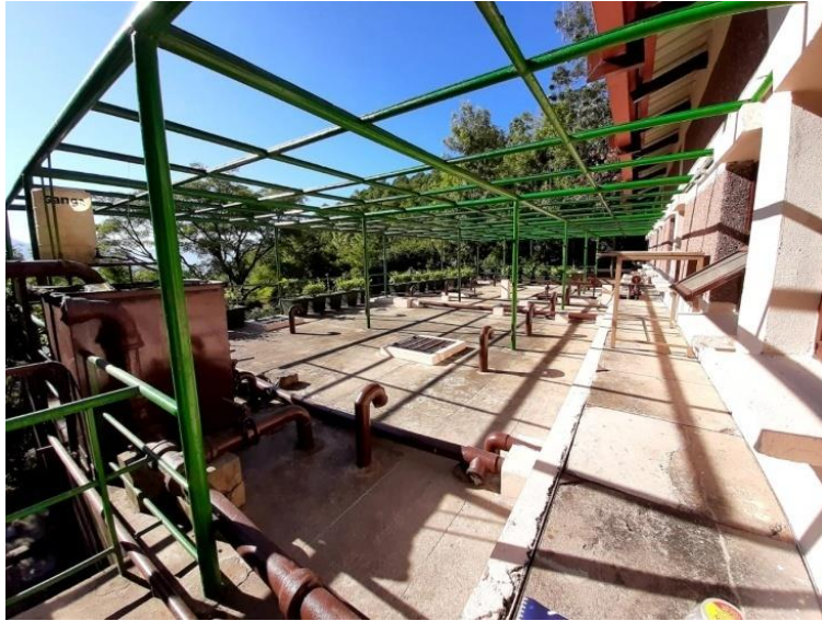
Figure 2: JUIT's Sewage Treatment Plant
