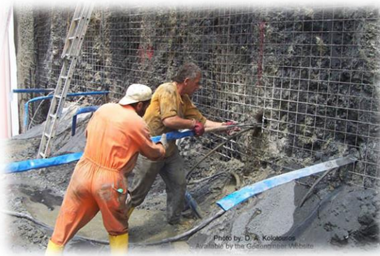
Fig 1.3: Grout is being placed with the help of pipes
