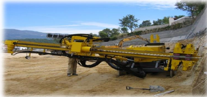
Fig 1.4: Typical drilling equipment
