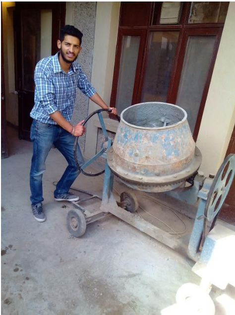
Mixing of aggregates
