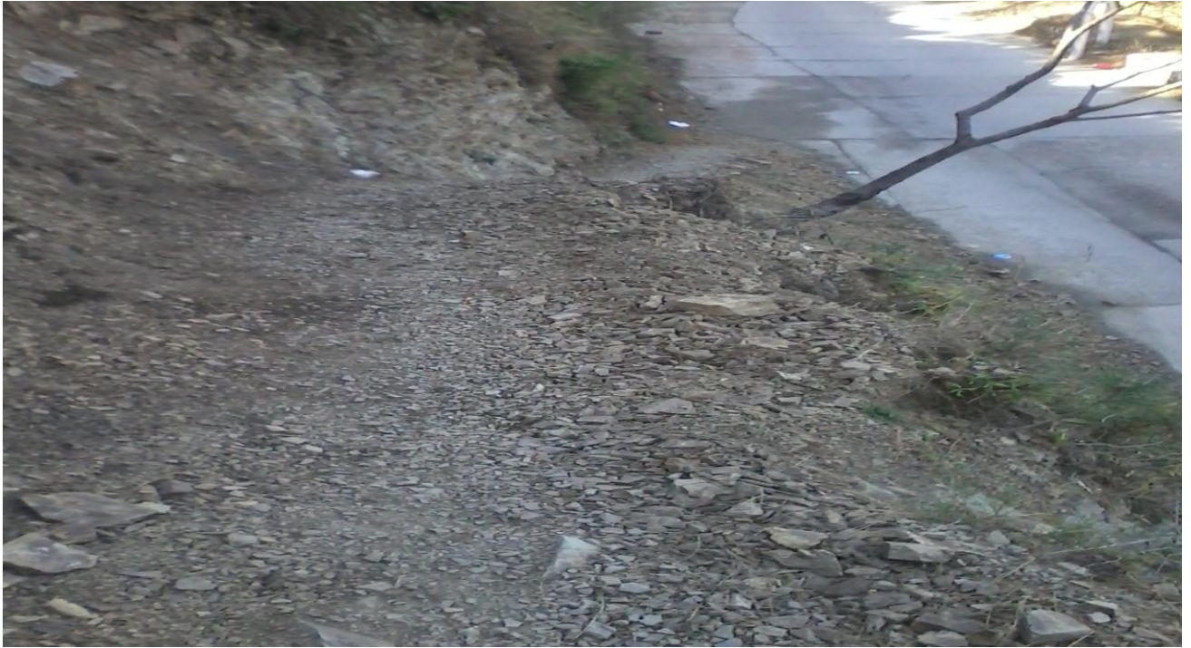
Fig 5.3(d) Condition of Tree is not good
