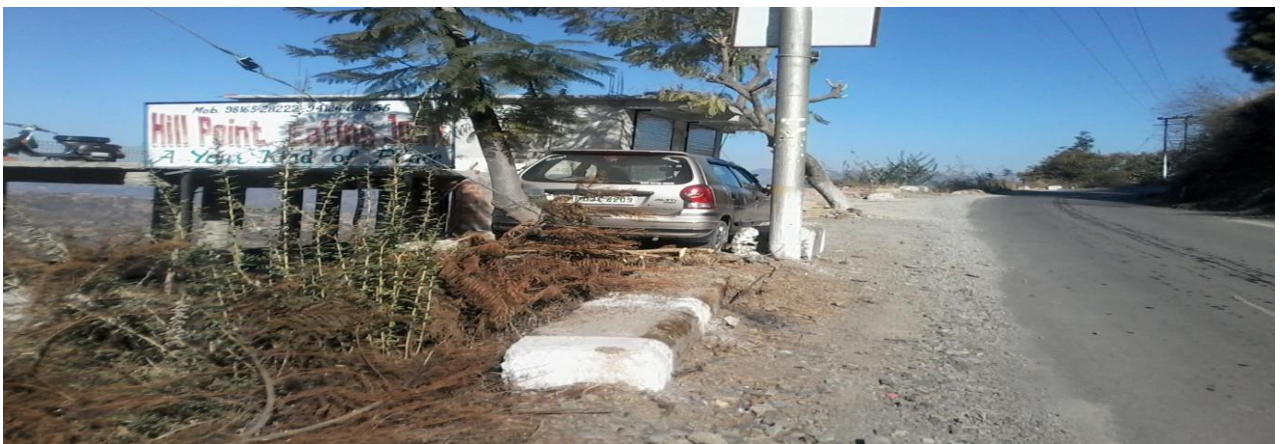
Fig 5.5 (b) View of Hill Point
