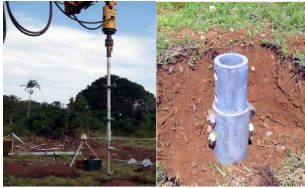
Fig. 1.2 Installation of helical pile foundation
