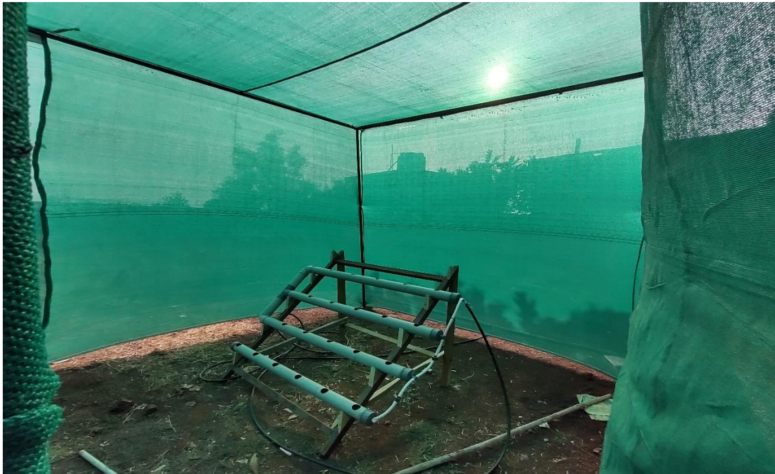
Fig.1 : Green net house constructed at home using Green net and Iron rods.
