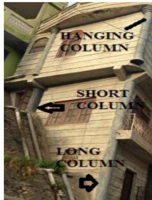
Fig 3.8 floating columns or short columns
