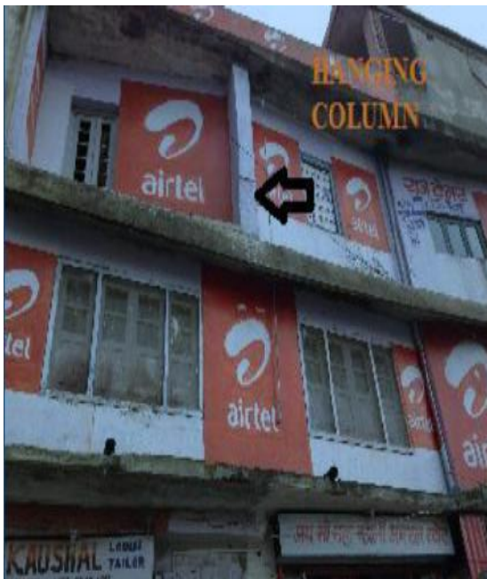
Fig 3.7 Hanging columns or floating columns
