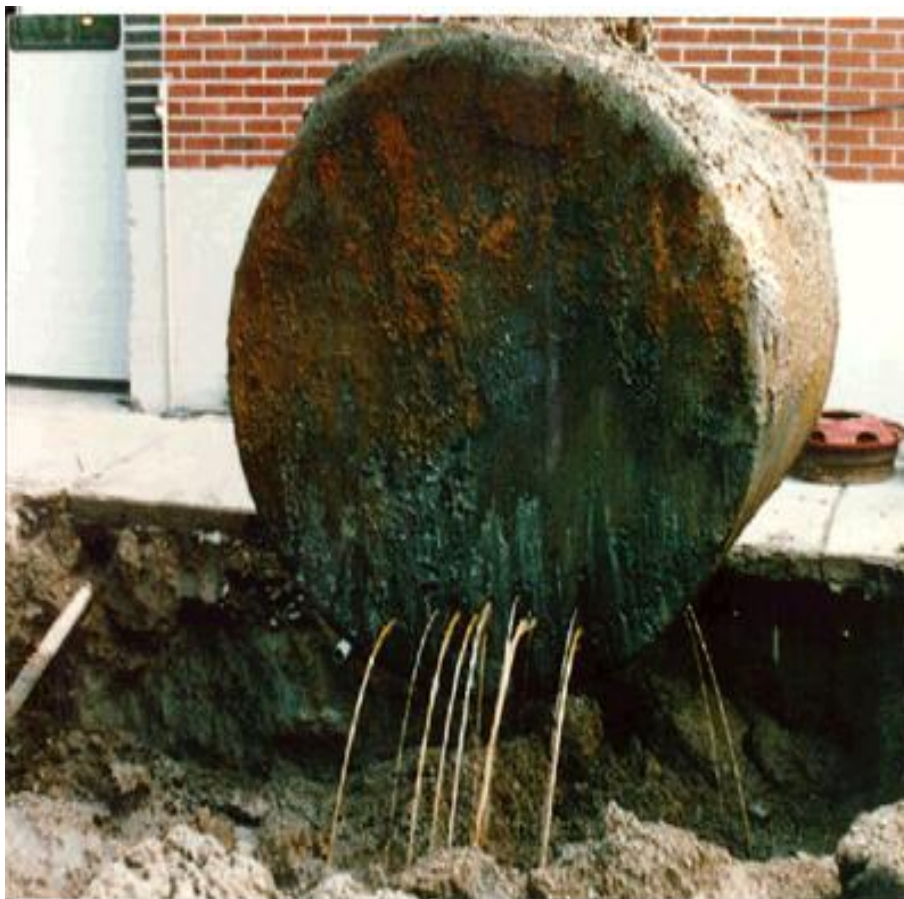
Figure 1.6 Leakage taking place in a tank [12]
