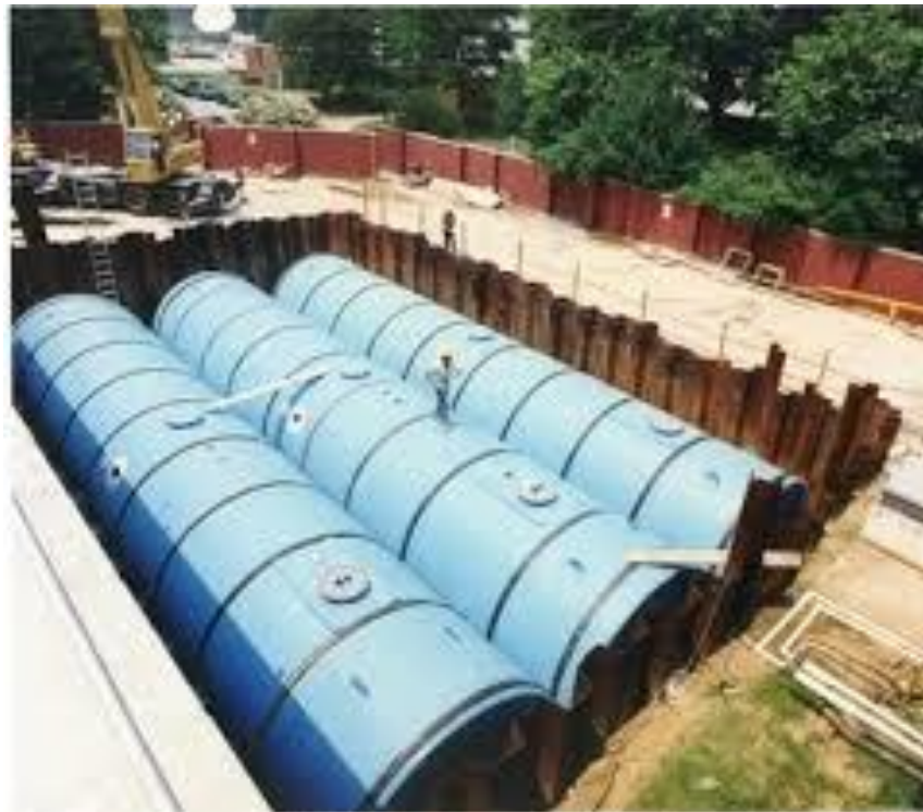
Figure 1.3 Underground Storage Tanks for holding various fluids [10]
