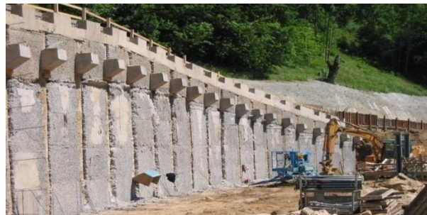
Fig.1.4 Bored pile retaining wall
