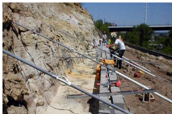
Fig.1.6 Anchored retaining wall
