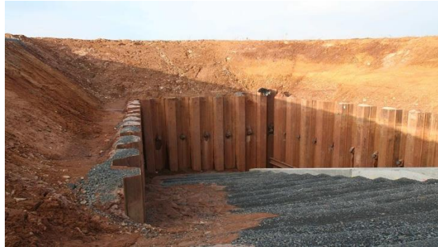
Fig.1.5 Sheet pile retaining wall
