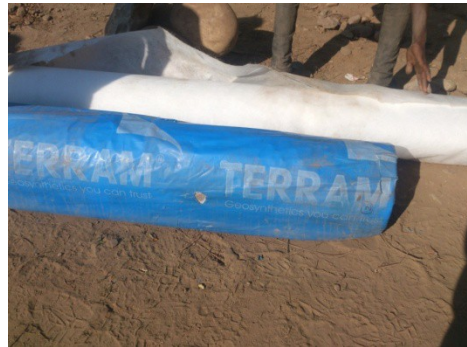
A roll of geotextile being opened at site
