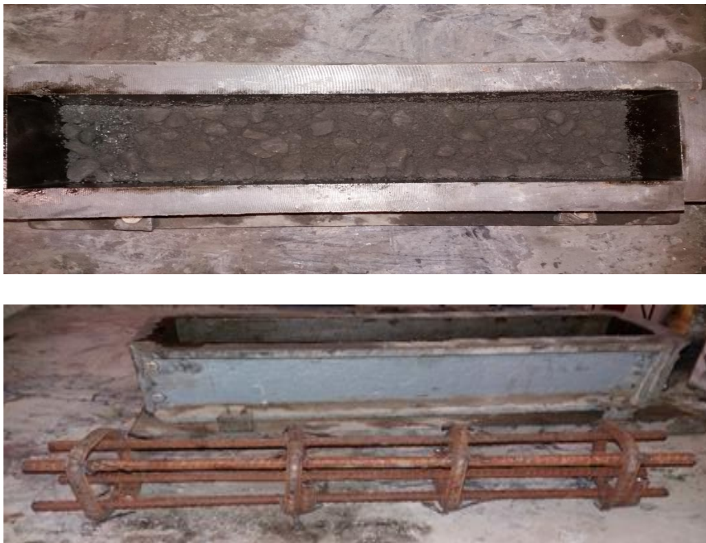
Fig 1: Casting of RCC Beams
