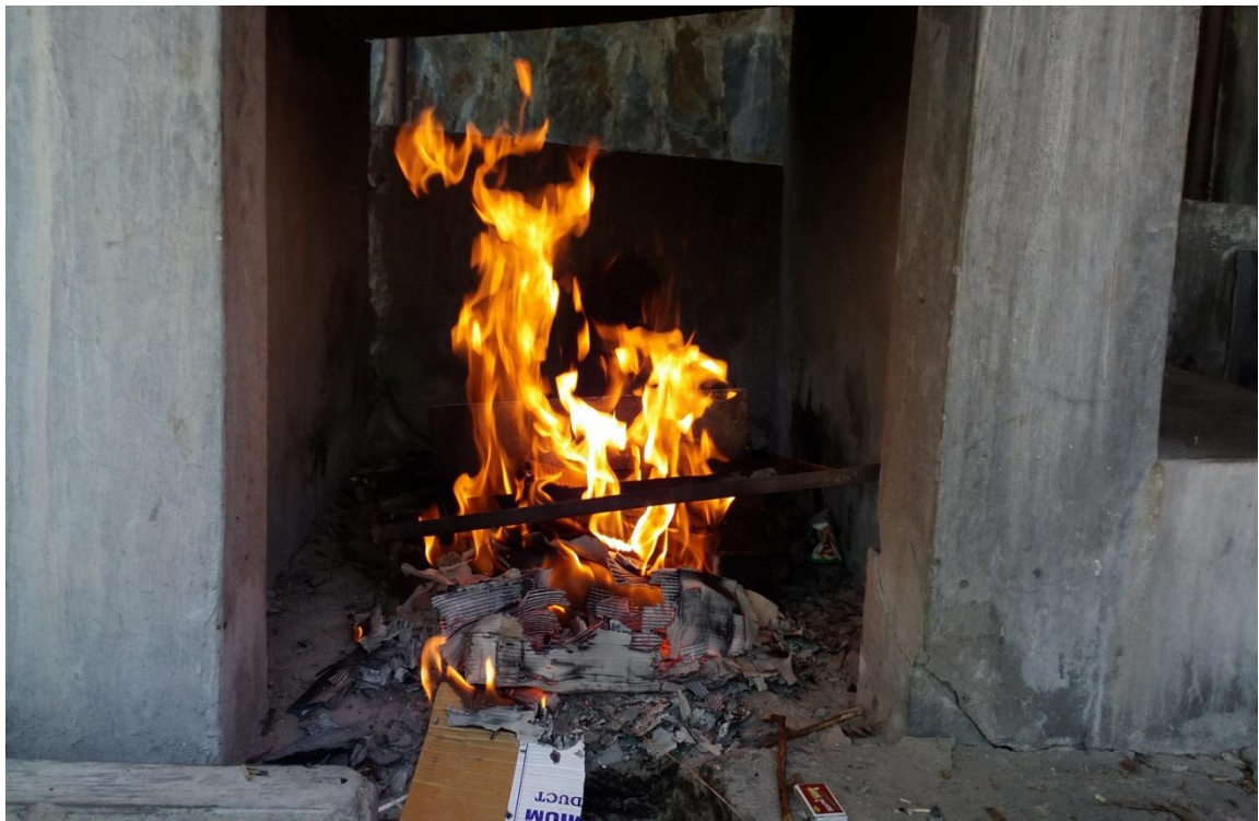
Fig 4: Burning of Beam
