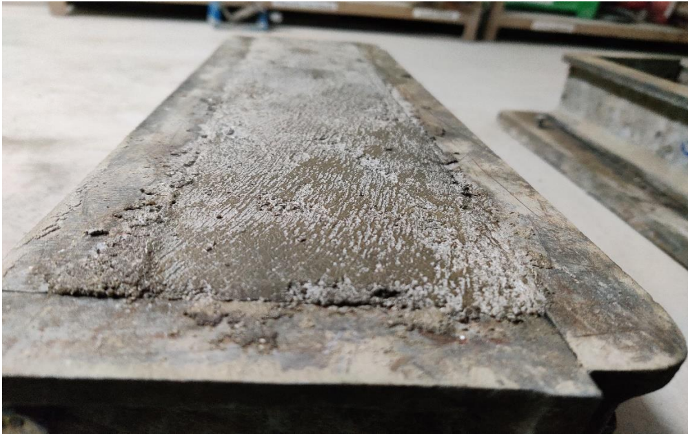
Fig 3.17 Casting of beam
