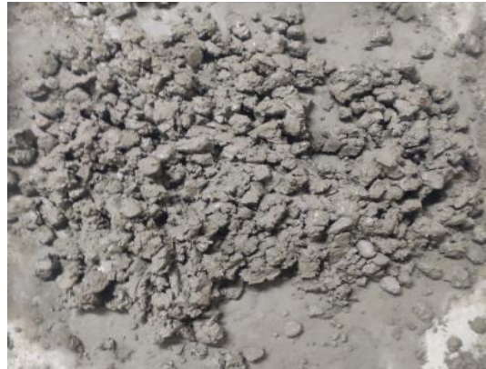
Figure 3.14: Preparation of concrete mix
