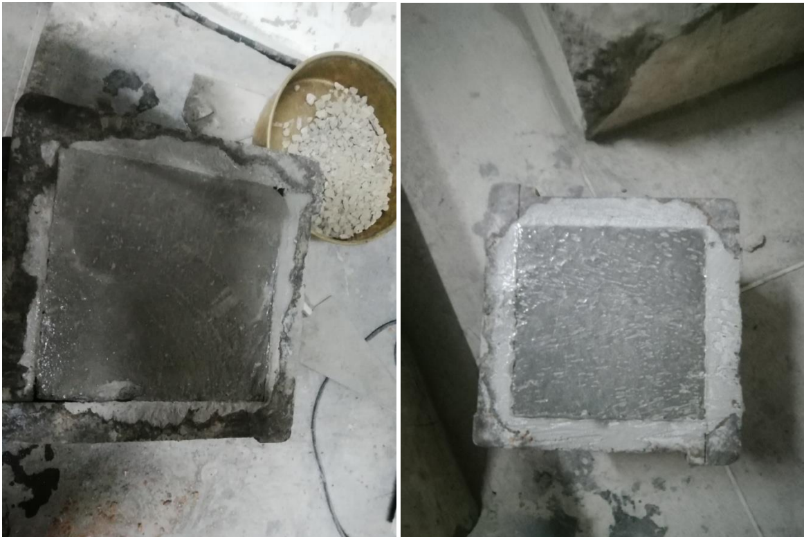
Figure 4.8: Casting of cubes
