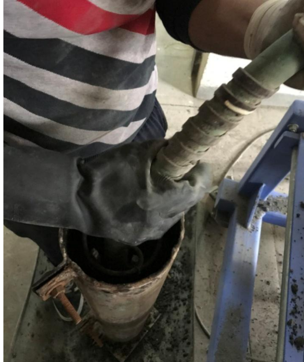
Figure 4.4 Compaction by needle vibrator while casting
