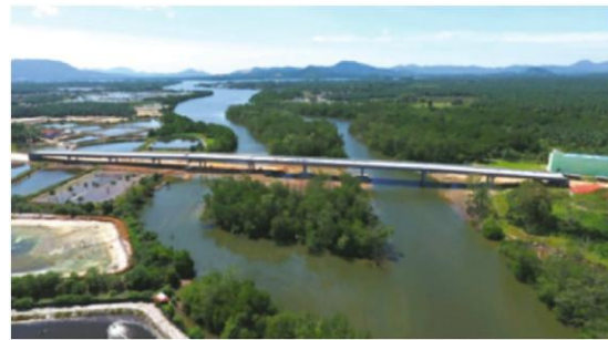
Fig. 2.6. Completed UHPC bridge in Malaysia [27].
