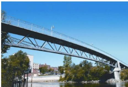
Fig. 2.5. Sherbrooke pedestrian bridge in Canada [22].
