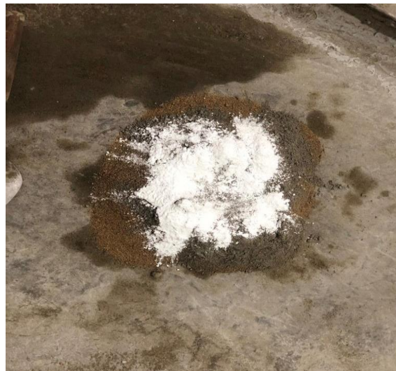
Fig. 4.1 Mixing Marble Powder, Cement & Sand.
