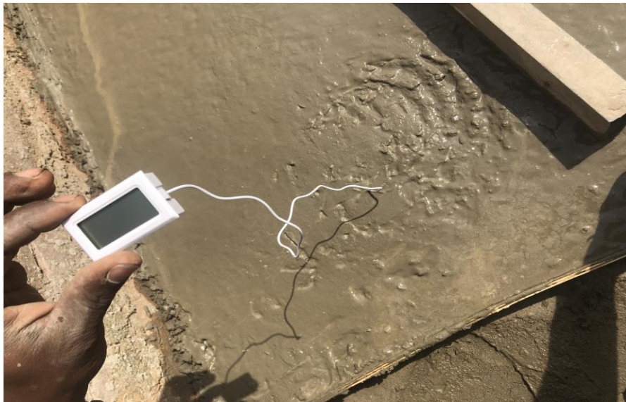
Fig. 4.7 Thermocouple used for measuring inner pavement temperature
