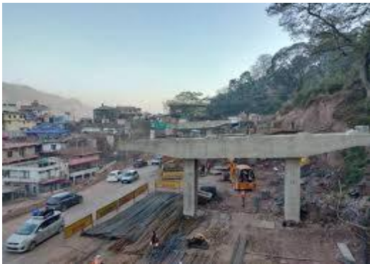
Fig.12. Construction of fly over
