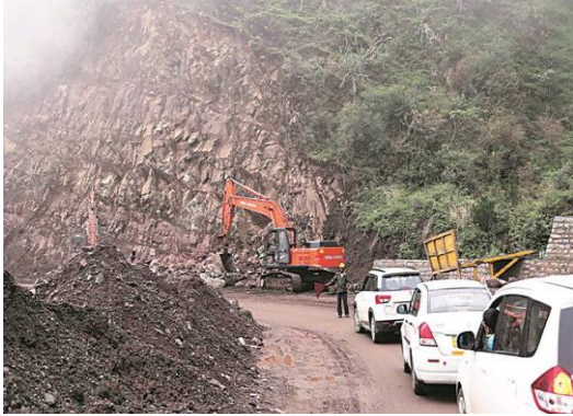
Fig.8. Cutting and levelling work
