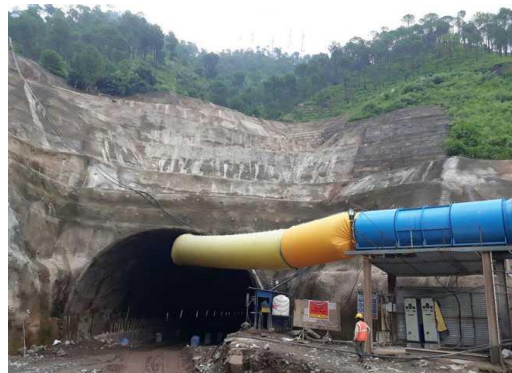
Fig.13. Construction of tunnel
