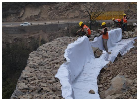
Fig.11. Installation of geo-synthetic
