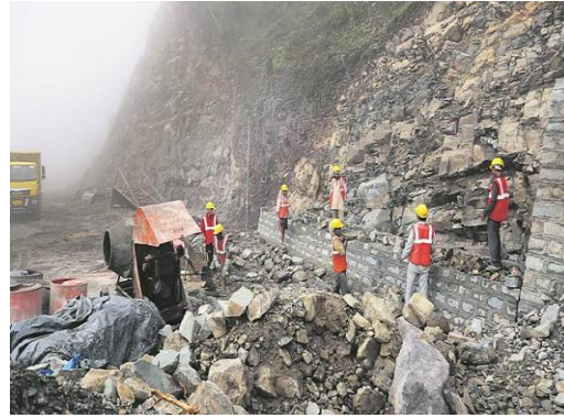
Fig.9. Construction of retaining wall
