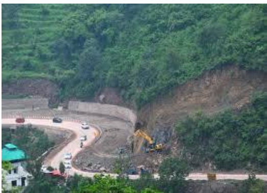
Fig.10. Preparation of levelled surface
