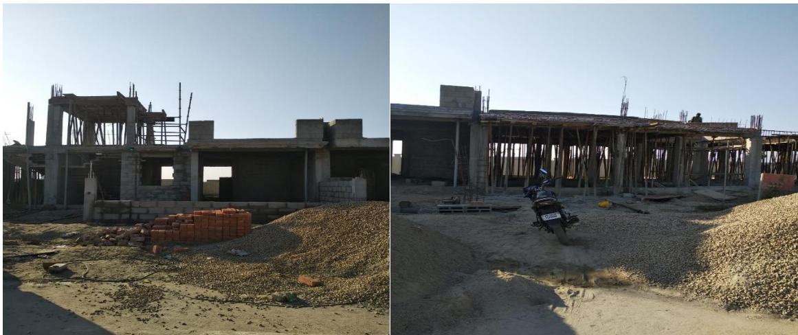
Fig 3.1: Construction of Villa in the Ludhiana GT road (Punjab)
