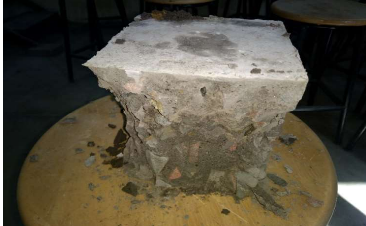
Figure-4 Concrete block after testing
