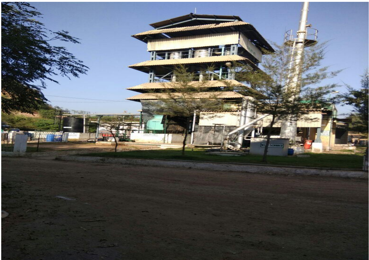
Figure 14 Location of Shivalik Solid Waste Management Plant
