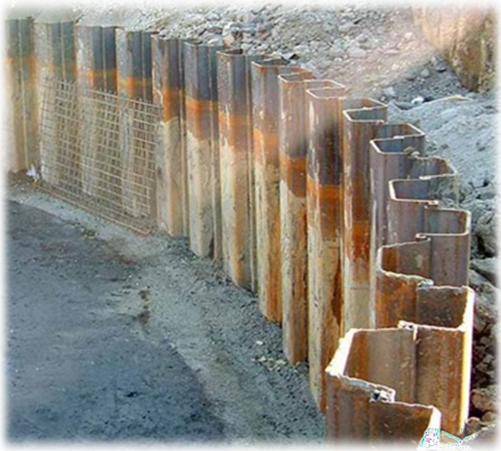
Fig 1.10 Sheet pile retaining wall
