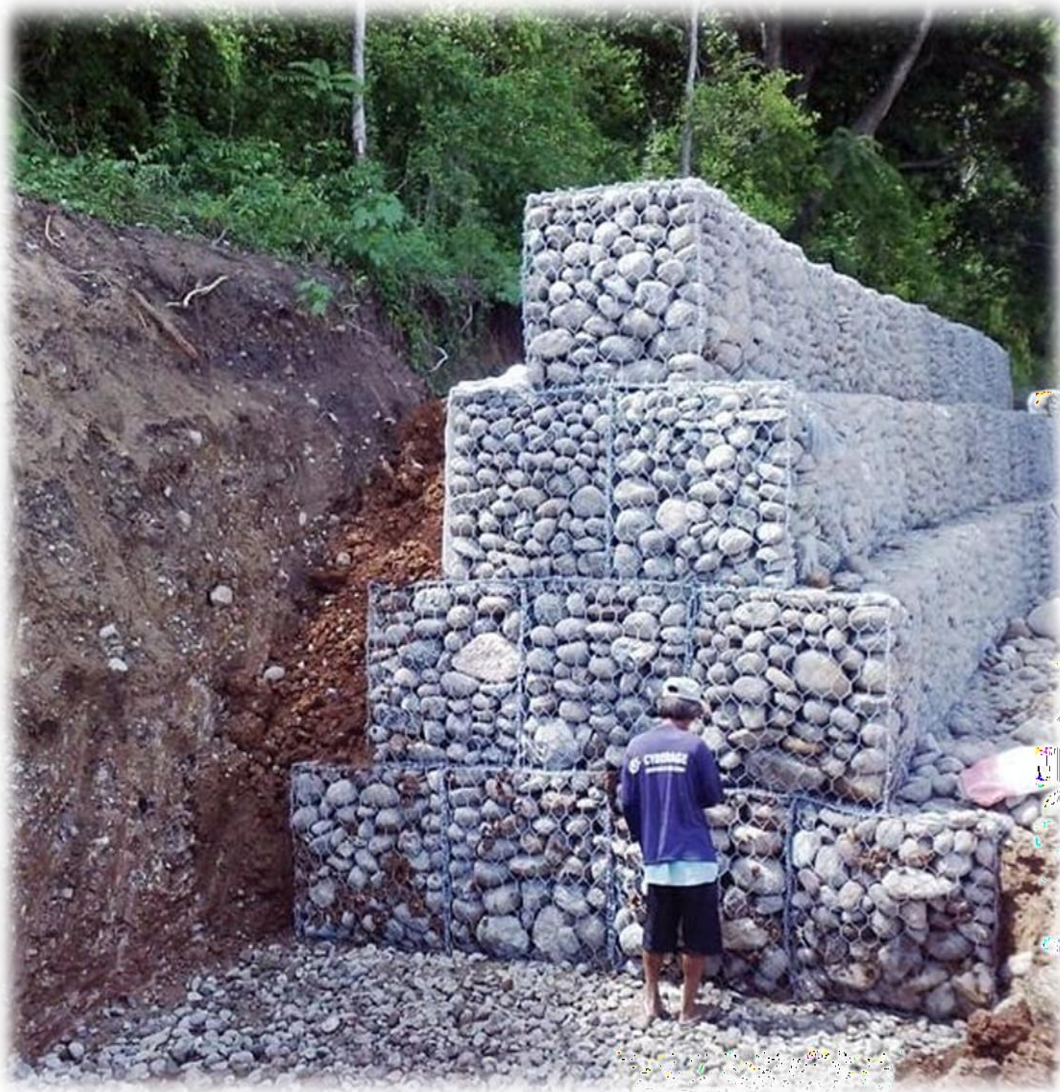
Fig 1.5 Gabion retaining wall
