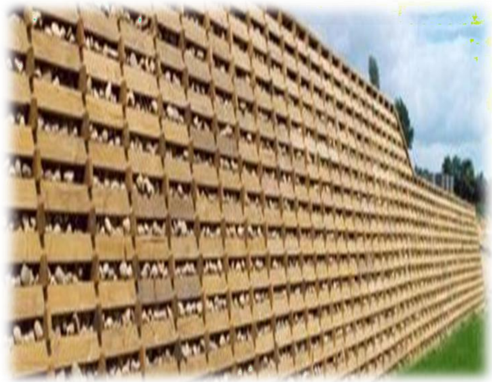
Fig 1.4 Crib retaining wall (a) and (b)
