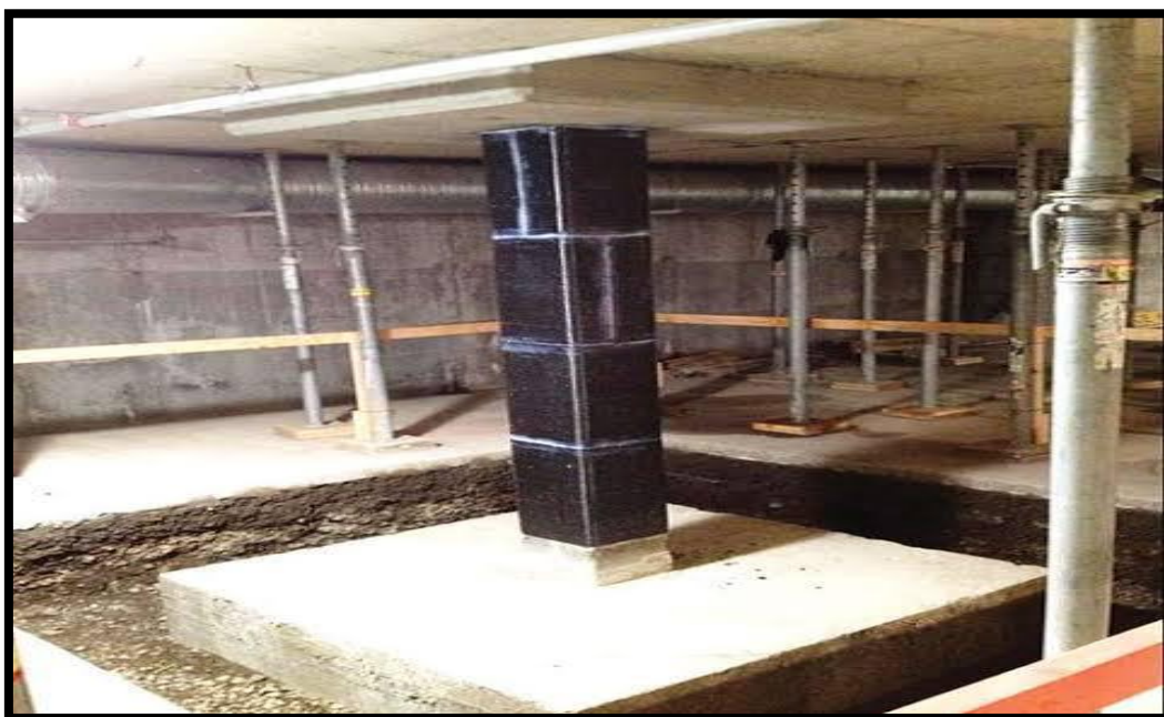
Figure 1.8: Retrofitting by Composite Fibre Wrap
