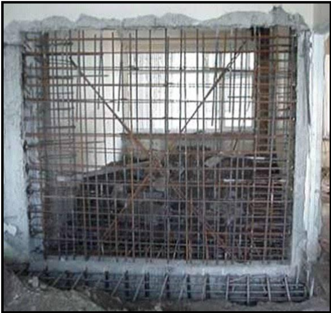
Figure 1.2: Seismic retrofitting by addition of shear wall
