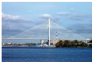
Fig.6 Cable Stayed Bridge
