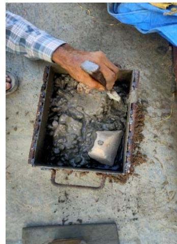
Figure 3.10: Filling gaps around stone with concrete
