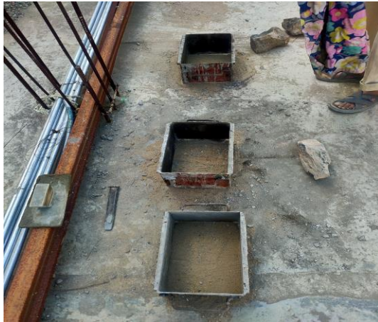
Figure 3.7: Moulds for blocks
