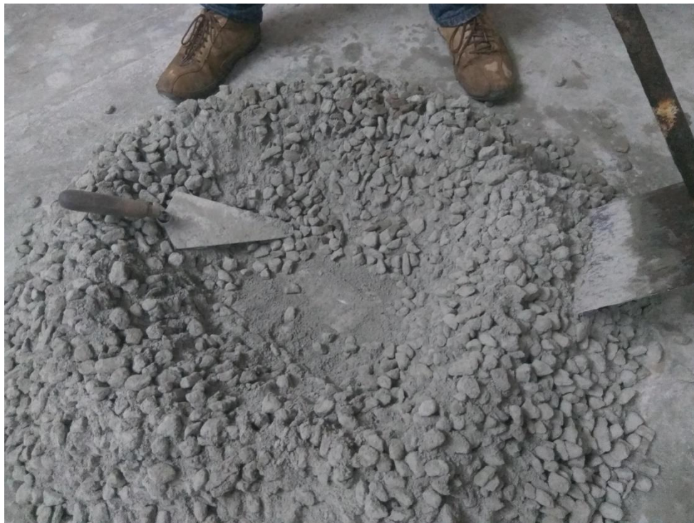
Fig 7.5.3.1: Homogeneous dry mix
