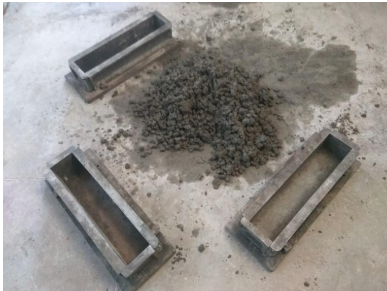
(A) Beam moulds prior to filling of concrete
