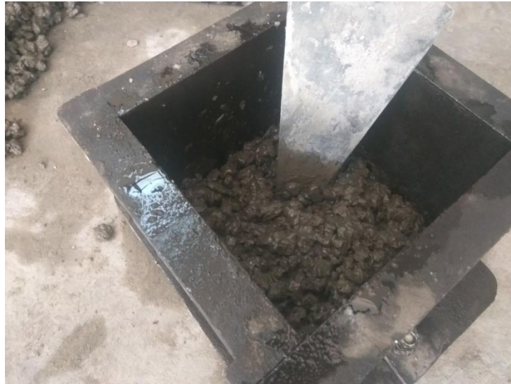
(B) Concrete filled in layers in cube moulds
