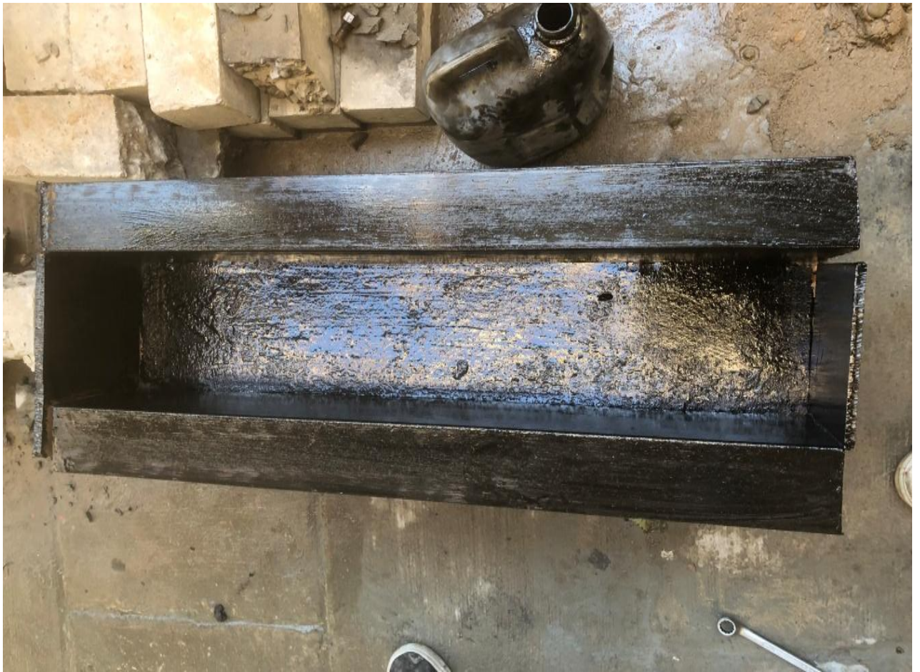
Figure 4.2 Oiling of moulds
