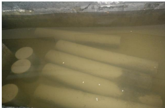
Fig3.5 Curing of Columns
