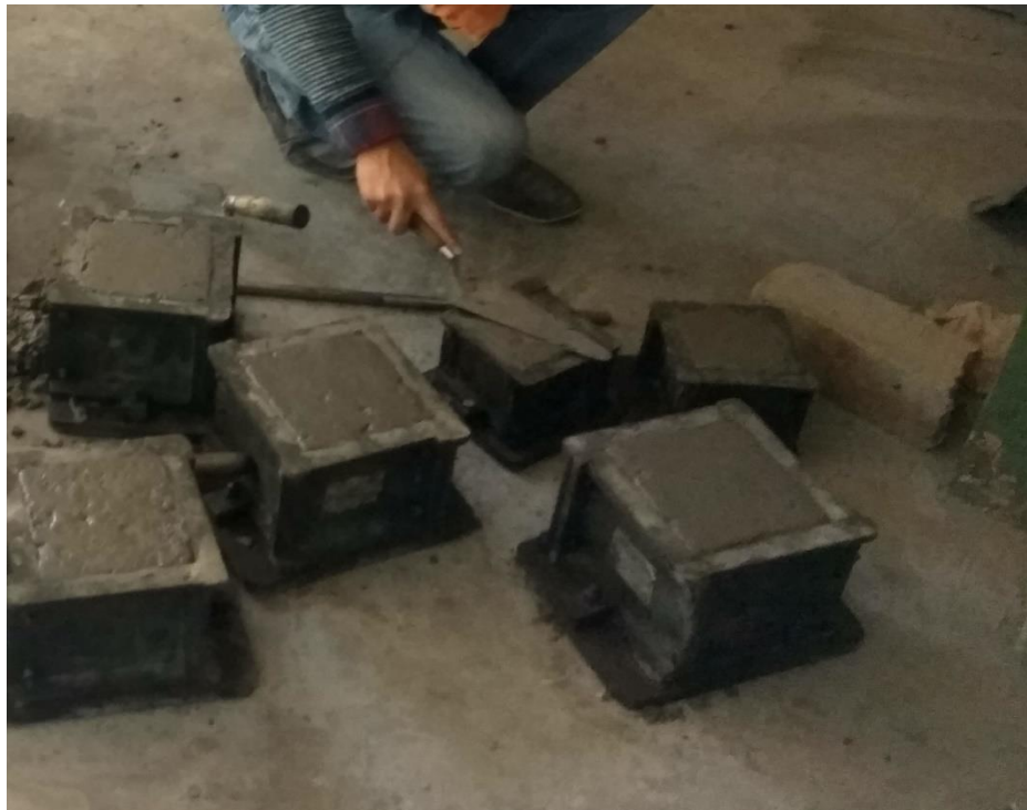
Fig 7.7: Levelling and finishing of top surface
