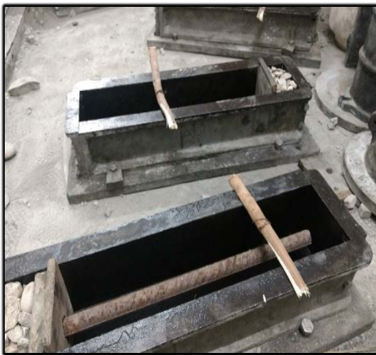
Figure 3.8: Preparation of moulds
